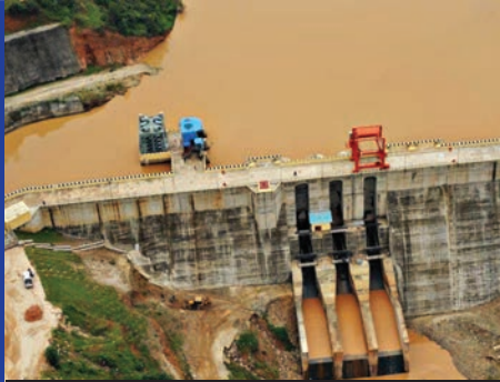
Nyabarongo, Hydropower, Rwanda
